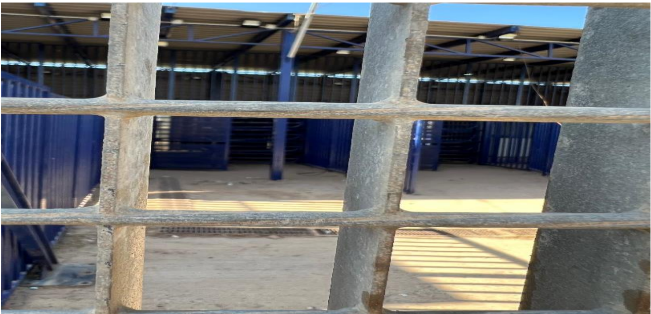
Picture 2 : Buffer zone where the revolving iron doors are located
